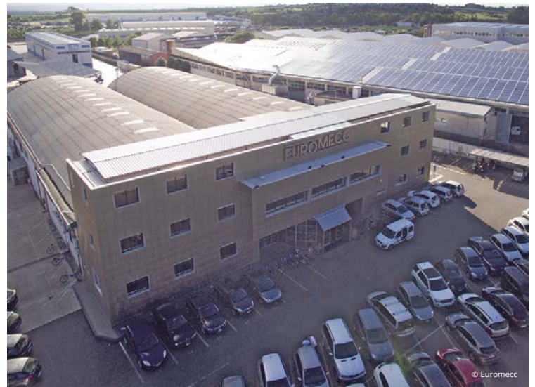
Euromecc's headquarters in Sicily (Italy) and, above, two of the storage terminals built by Euromecc.
