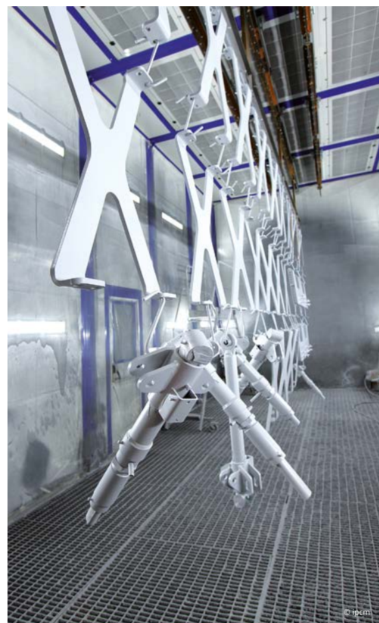
Powder top coat application in one of the two dedicated booths.
